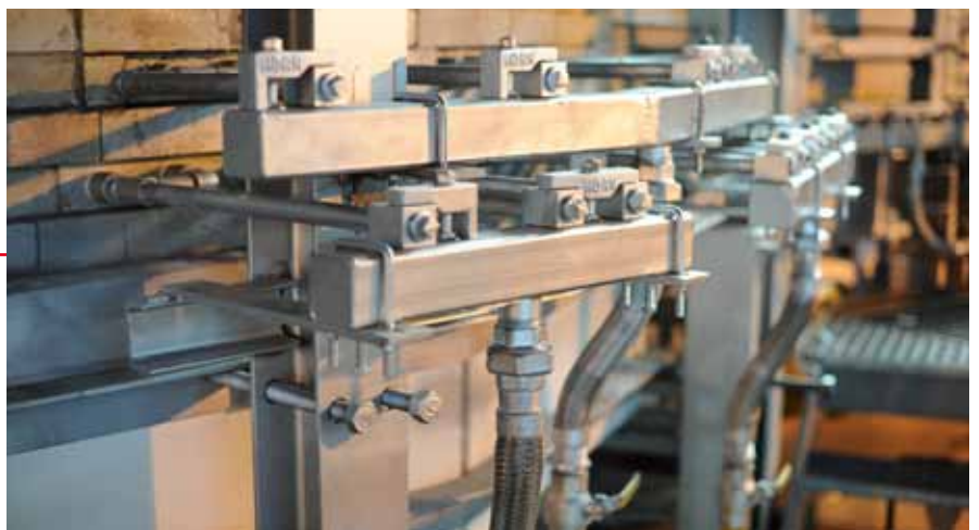
Double burner manifold Gas / air mixture burners
